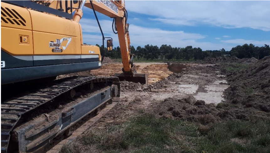
Above: earthworks for the foundations of the Class C to Class B treatment plant
