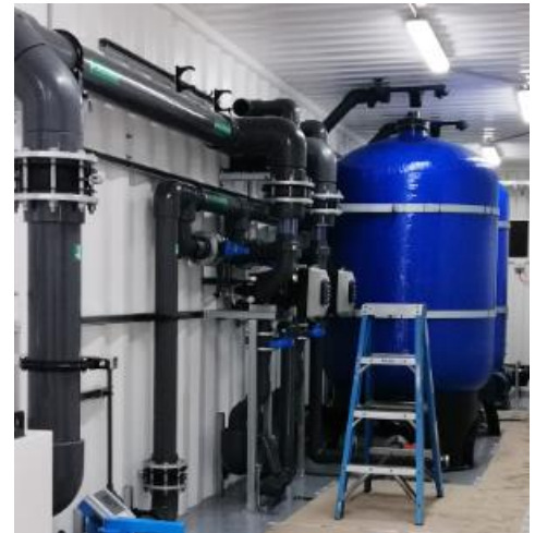
Above: part of the C to B treatment plant
