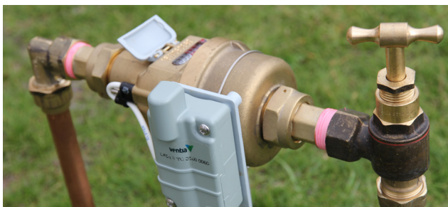
Above: The digital data logger device attached to an existing customer water meter.
