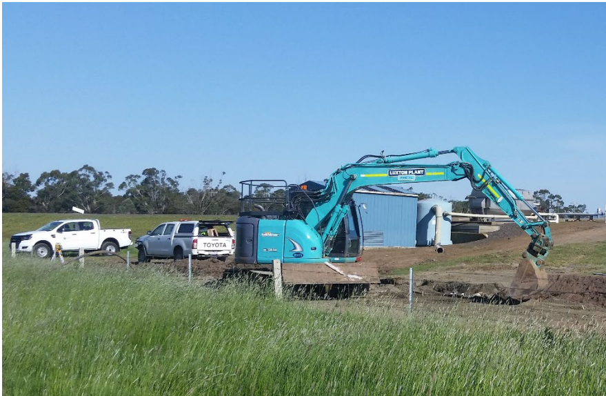
Groundwork for three 30 kilolitre tanks to supply irrigation water to Hardwick's
