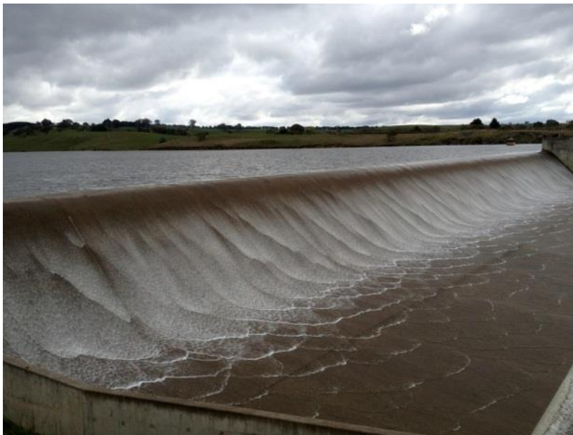
Figure 2: The Upper Coliban Reservoir spilling in September 2013
