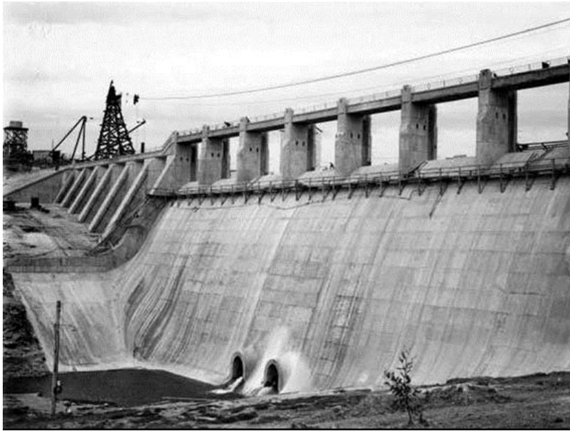
Figure 3: Lauriston Reservoir under construction in 1940s
