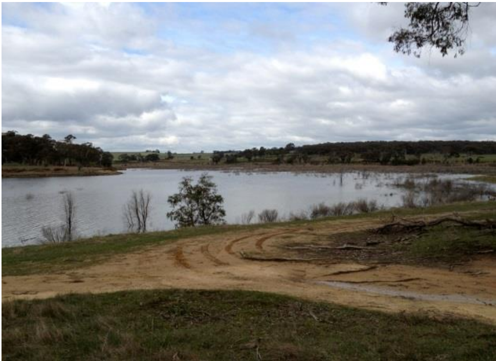
Figure 7: Southern end Malmsbury Reservoir approaching full supply in spring 2013.
