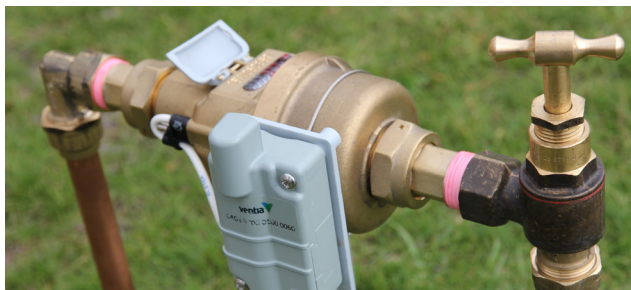
Above: The digital data logger device attached to an existing customer water meter.
