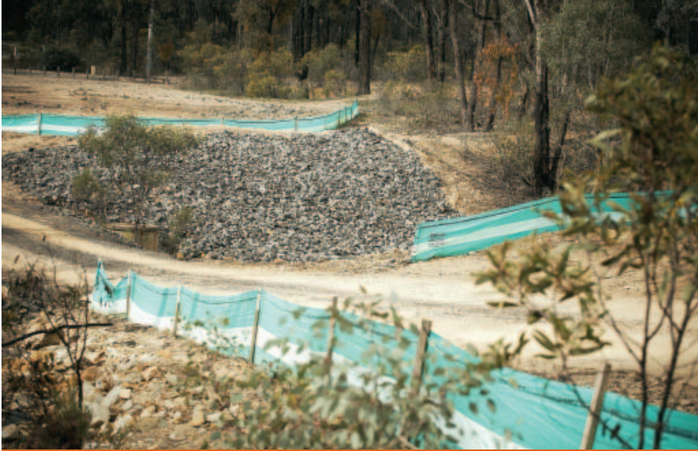
Environmental silt fencing, Eppalock to Sandhurst Augmentation Project
