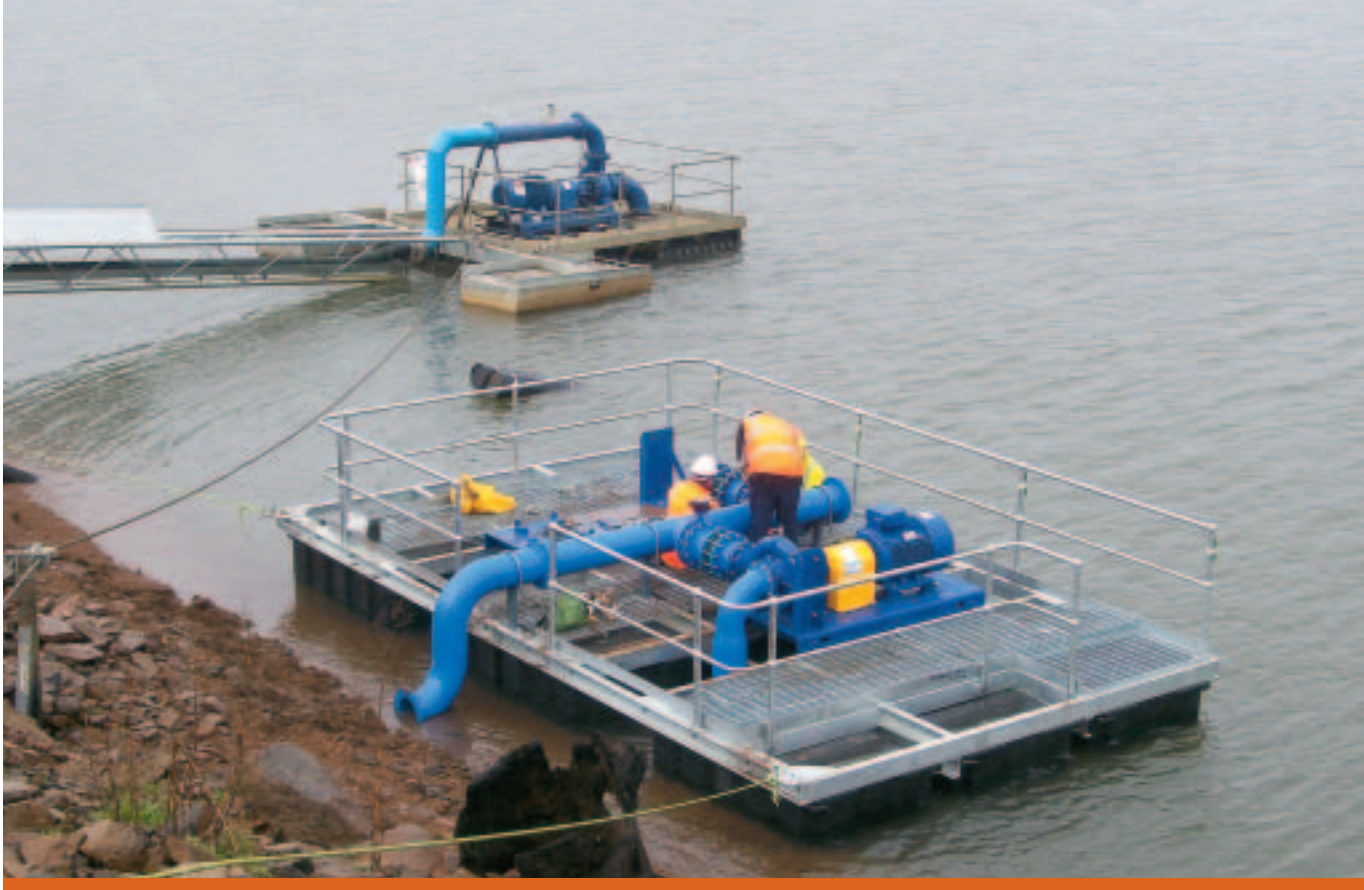
Construction of pontoon mounted pumps at Lauriston Reservoir
