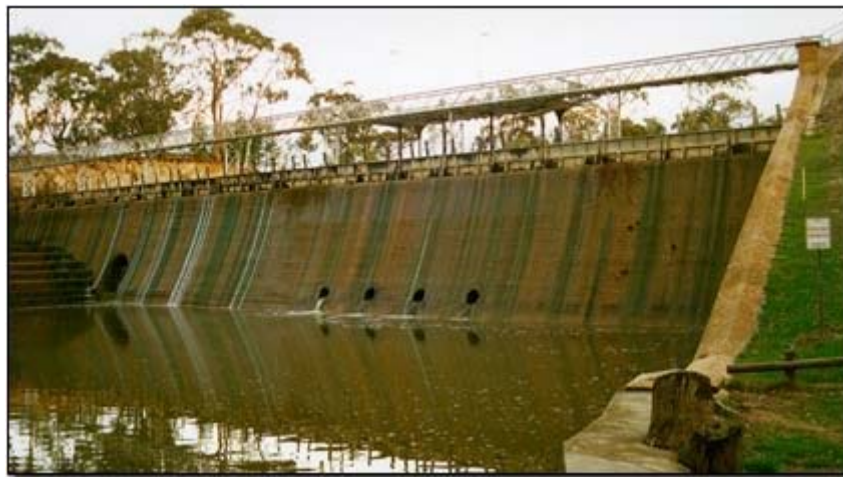
Laanecoorie Reservoir, Loddon River, completed 1891
