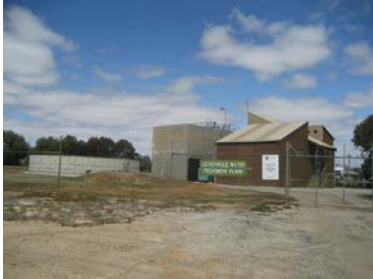
Leitchville Water Treatment Plant.
