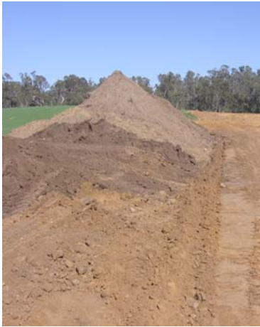
Example of how topsoil will be stockpiled for the reinstatement phase
