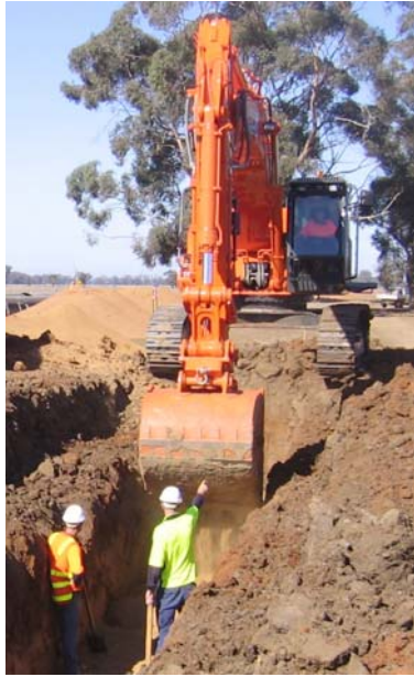
Contractors working on new pipelines in the Bendigo region
