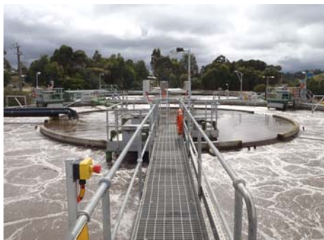
Above: Recommissioning of Demand Aeration Tank, April 2011.
