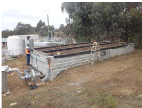
Above: Biofilter installation, May 2011.
