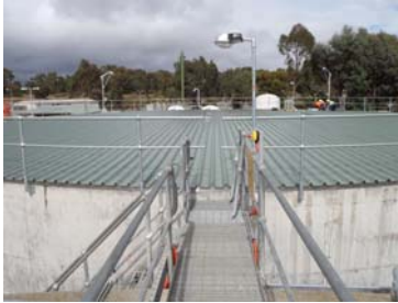
Above: New cover to Anaerobic Tank, April 2011.
