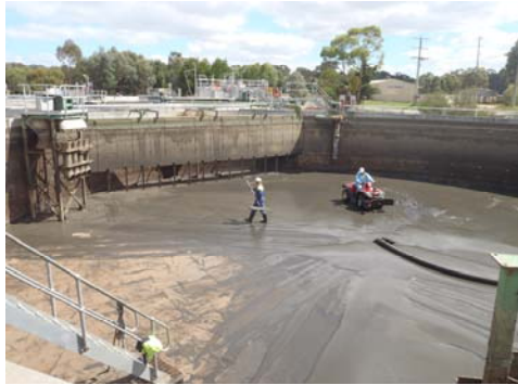
Above: sludge cleaning of Intermittent Aeration Tank, March 2011.
