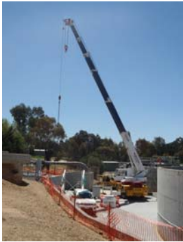
Above: Crane erecting inlet structure at CWRP, October 2010.
