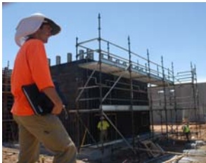
Above: Bendigo Recycled Water Factory during construction.
