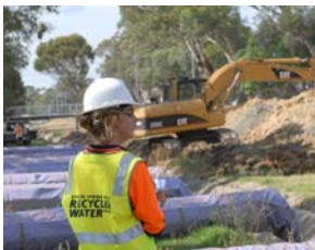
Below: Epsom to Spring Gully Pipeline during construction.
