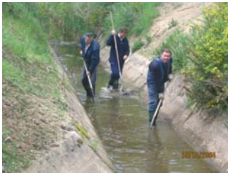
Channel maintenance works.
