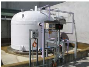
Recycled Water Factory, Bendigo Water Reclamation Plant, Epsom
