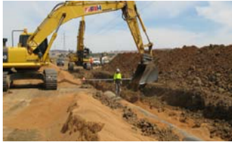
Goldfields Superpipe construction underway
