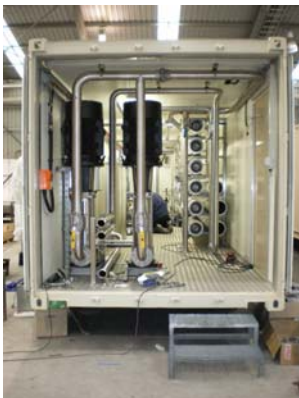
Above: Salinity Reduction Plant construction for Bridgewater June 2009.
