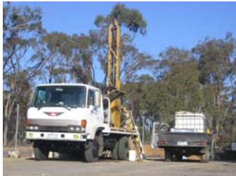
Above: Groundwater drilling at Laanecoorie June 2009.
